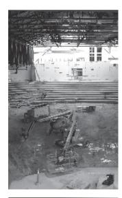
(Above) Inside the new Crownridge Campus Worship Center, concrete pours for the elevated seating, and main stage have been completed. The roof structure is in place, with each support crossbeam measuring 120 feet long and weighing 70 tons.
